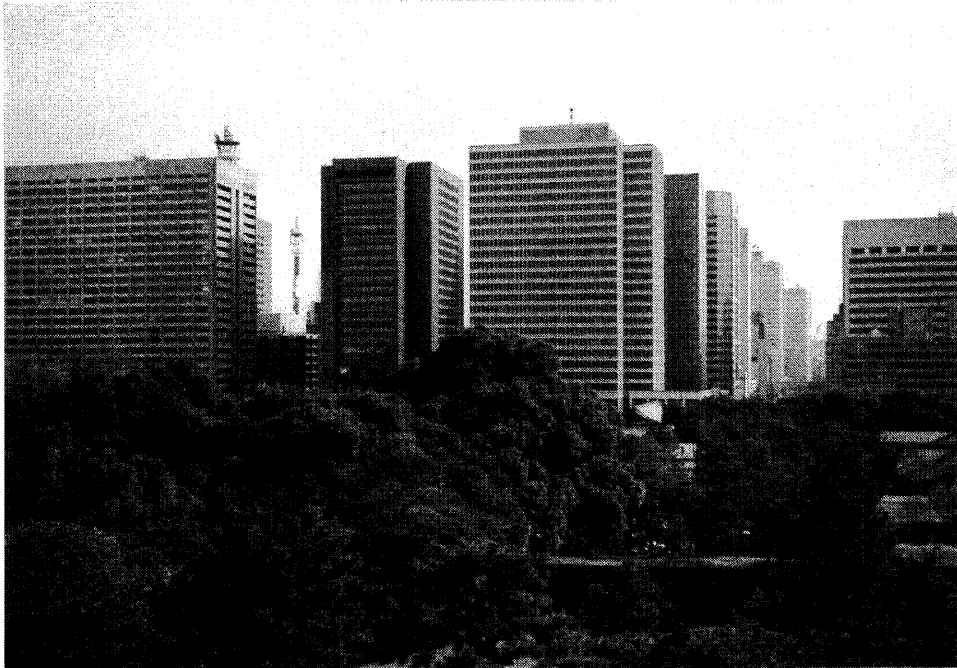
Photo 10 Buildings with same eaves height (100m) in Otemachi district (1993).
