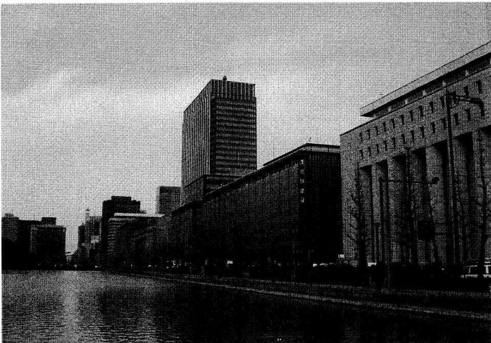
Photo 8 Buildings with same eaves height (31m) in Marunouchi district (2004).
